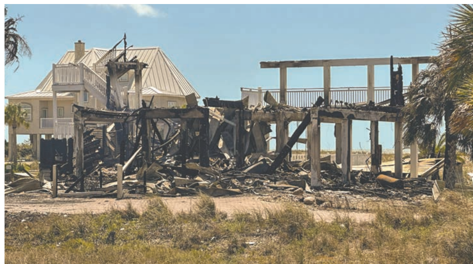
The house at 1136 East Gulf Beach Drive was left with little more than charred bones. [ OYSTER RADIO | CONTRIBUTED ]
